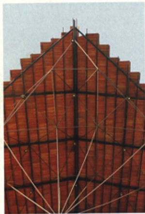
The cantilevered roof shields the structure from the vagaries of the weather
